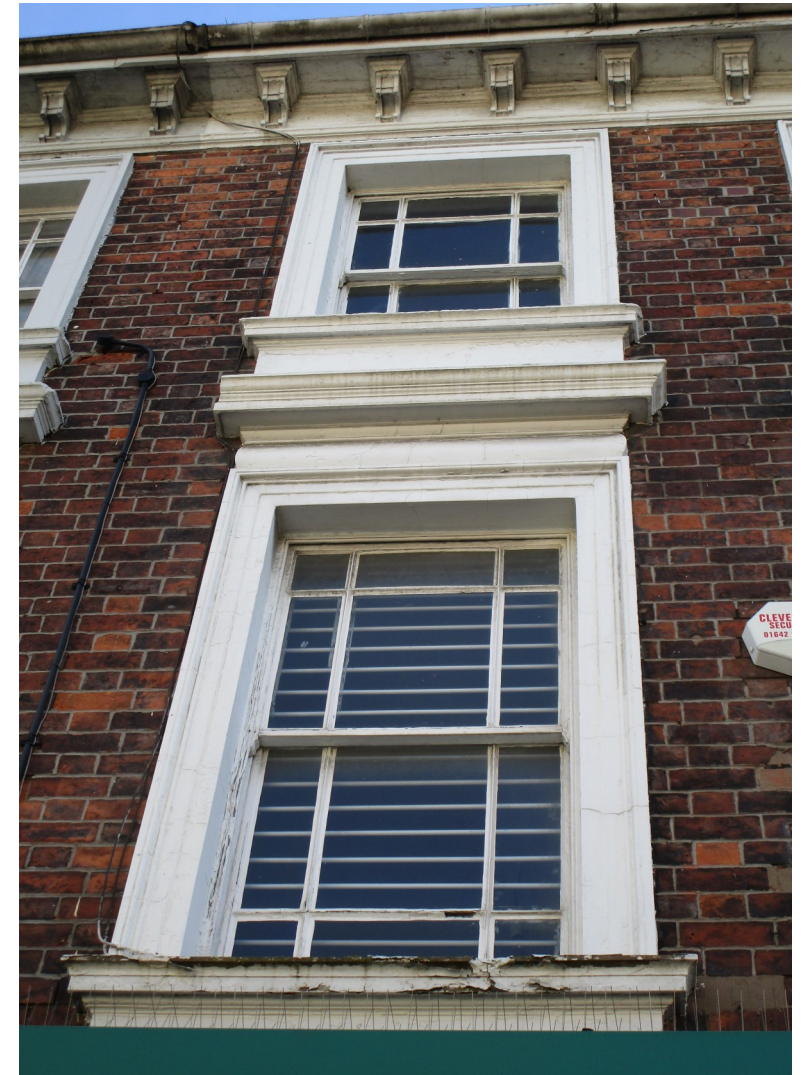
Plate 41 No. 342-345 High St, detail of a 1 st and 2 nd floor sash window with margin lights, the 1 st floor painted stone window surround is topped with a cornice, and the eaves are bracketed. The brickwork is in Flemish bond.
